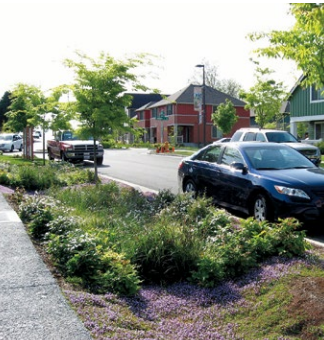
Example of pervious pavement (left in photo) and a street-side swale in Seattle's High Point neighborhood. Courtesy Green Infrastructure
