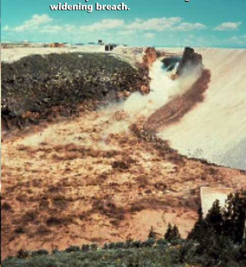
Water spills unchecked through the widening breach.
