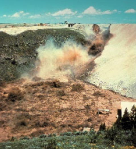
The dam is breached.
