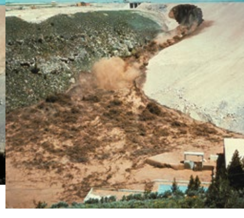
The hole in the dam face continues to enlarge upward near the crest of the dam, the rush of water increases markedly, and erosion cuts deep into bedrock of the abutment.
