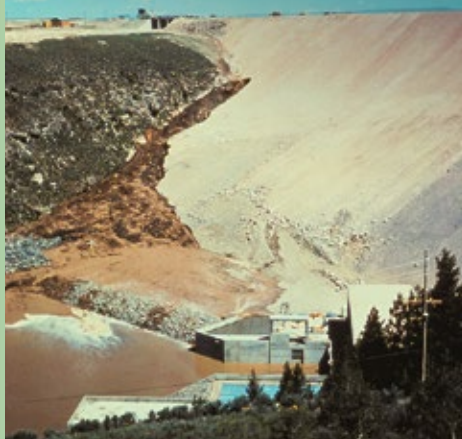
View northwest toward the right abutment of the Teton Dam. Muddy water issues out of the hole about two-thirds up the face of the dam and begins to pond at the toe.
